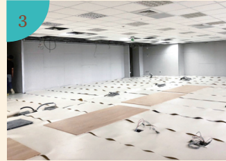
Install Plyboard
