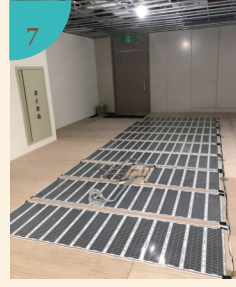
Complete installation of heating membrane
