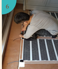
Heating membrane installation
