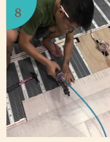
Laying of wooden floor with blind nails
