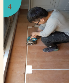
Forming of cable trenches
